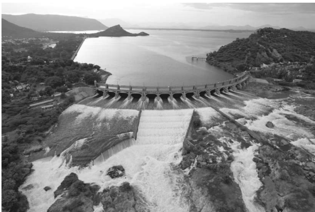
Fig. 2. Mettur Dam, Salem District
